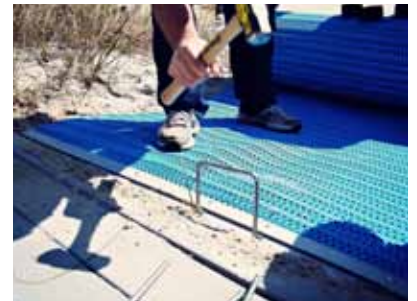
Pinning down the ends
